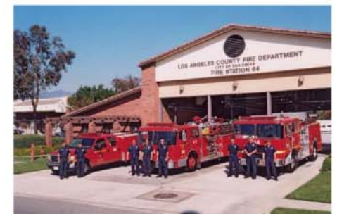
A Fire station
